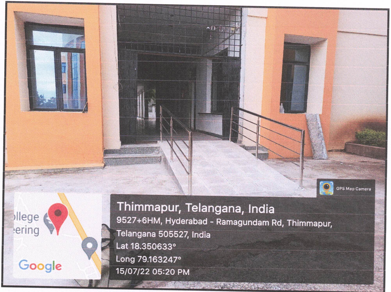
Ramp at main entrance
